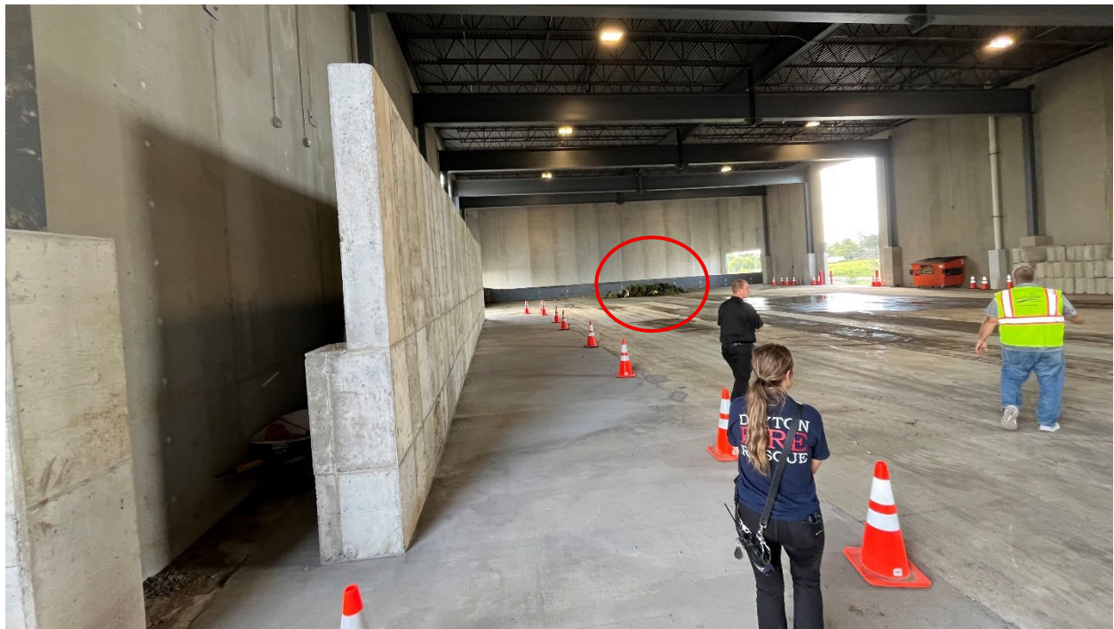
Curbside Transfer Station. Yard waste (circle) is trucked into the building and dropped on the floor. If additional types of wastes are added, Curbside would build bins against the push wall (left) for dropping. Then transfer waste from the bins into trucks (photo Jul 3, 2025).
